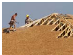
In this photo taken July 15, 2011, carpenters work
